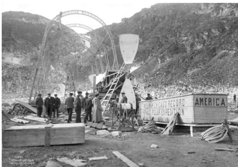
Figure 7 The hangar and airship under construction, Virgohamna, 1906. The person standing in front of the propeller blade is most likely Walter Wellman. (Courtesy Norwegian Museum of Cultural History [Norsk Folkemuseum].)
