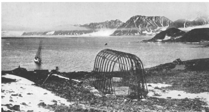
Figure 11 The hangar, rebuilt for the 1909 expedition with nine supporting arches, and without the diamond-shaped supports made by Liwentaal in 1906. (From Wellman 1911.)
