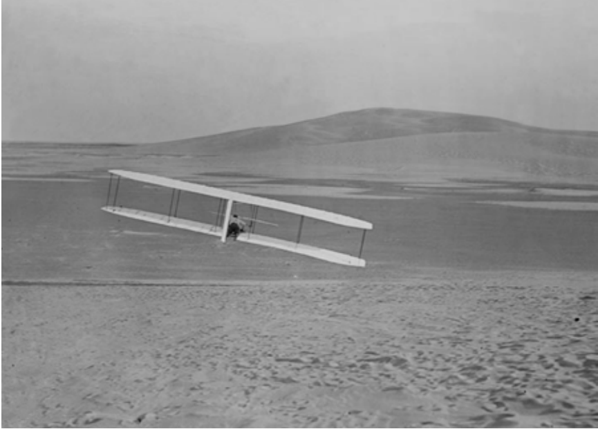
Wilbur Wright makes a right turn in the 1902 glider. The three-axis control system made this craft the world's first fully controllable flying machine. (Library of Congress)
