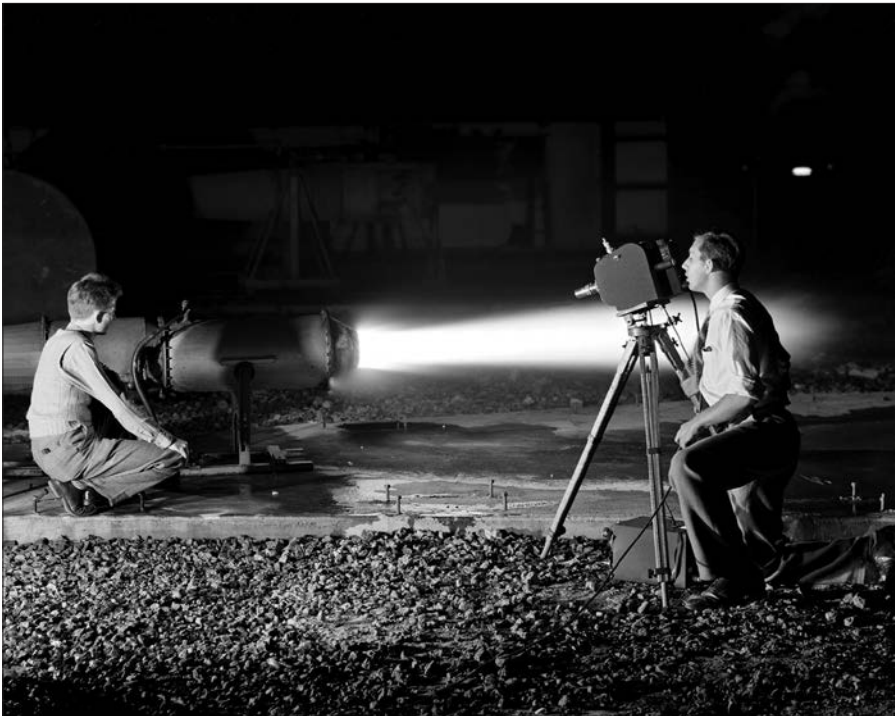
Figure 4-3. This 1946 test of an I-40 Ramjet engine at the NACA’s Flight Propulsion Laboratory in Cleveland measured the exhaust gases being discharged from a special burner. Engineers record the test with a motion picture camera. (NASA, GRC-1946-C-16086)
