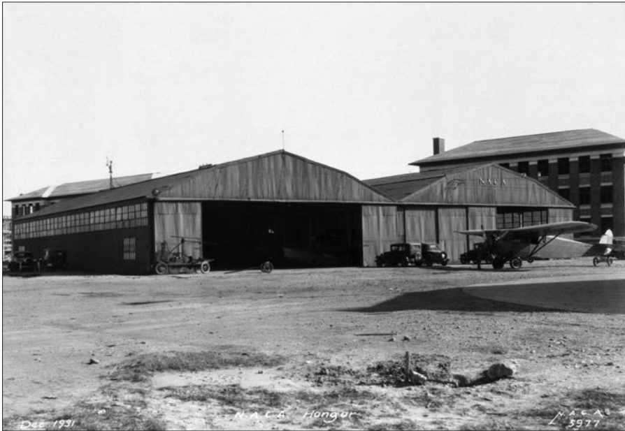
Figure 2-1. These hangars at the Langley Memorial Aeronautical Laboratory were some of the first structures built by the NACA. This image from 1931 shows a Fairchild test aircraft as well as a modified Ford Model A that was used to start aircraft propellers. (NASA, LRC-1931-B701_P-05977)
