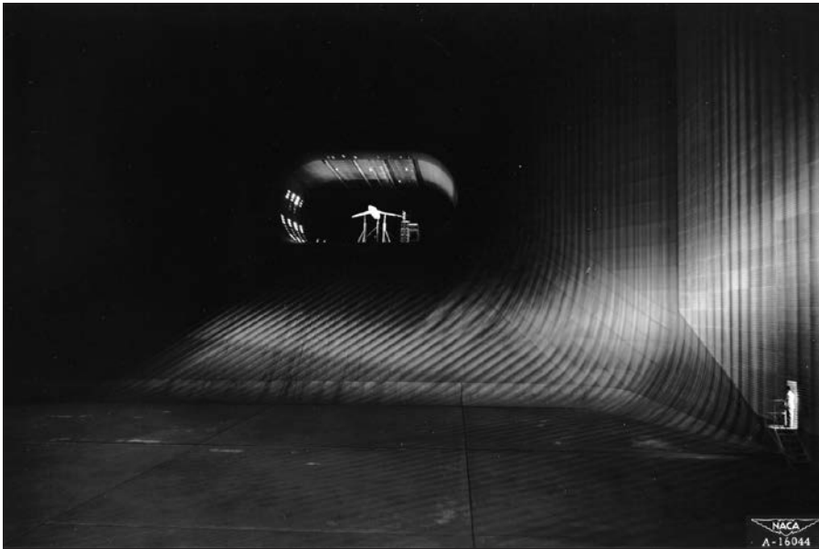
Figure 3-2. The NACA's Ames Aeronautical Laboratory in the Bay Area featured the largest wind tunnel of the agency, the 40- by 80-foot tunnel. This 1947 photograph shows a test aircraft dwarfed by the tunnel's massive size. (NASA, A-16044)
