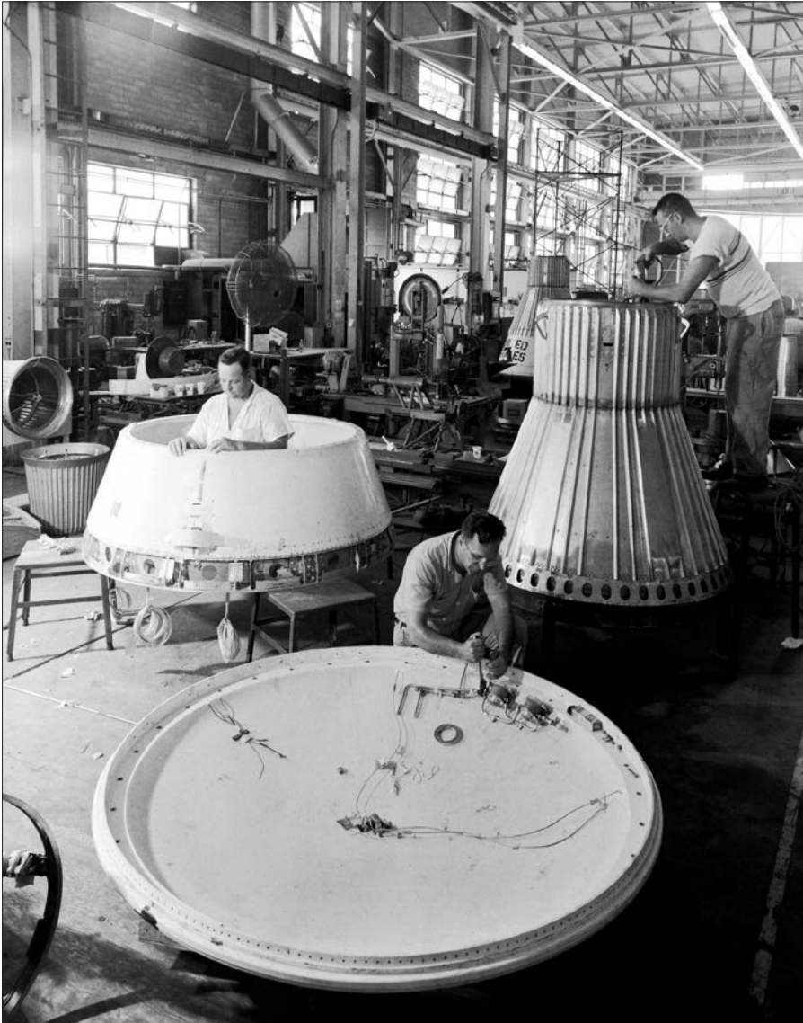
Figure 5-2. NASA technicians assemble Mercury Little Joe boilerplate capsules designed to launch monkeys. The bulky test equipment and a less-than-sterile environment are a far cry from the clean-room conditions that emerged in Project Apollo. (NASA, LRC-1959-B701_P-04947)
