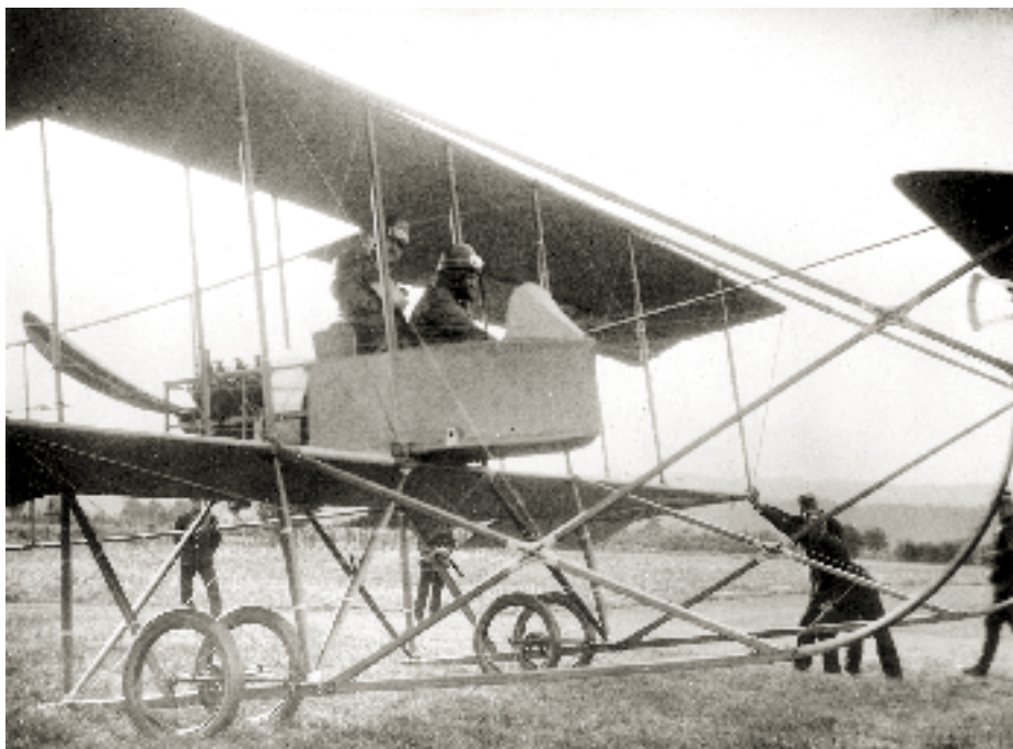
(Over) The first Army aircraft type, the Farman Longhorn, approx. 1912. The propeller was placed at the back, pushing the airplane forward.
