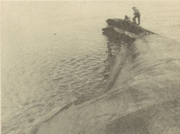
VIEW OF BOW DAMAGE BY 12,000 lb. BOMB HIT APPROX. 100 ft. DESTROYED
