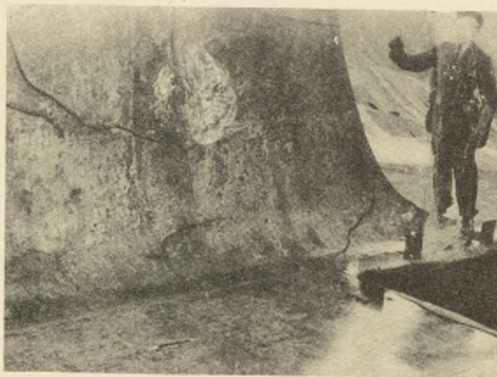
CRACKS IN STARBOARD SHAFT HOUSING FROM MIDGET SUBMARINE ATTACK
