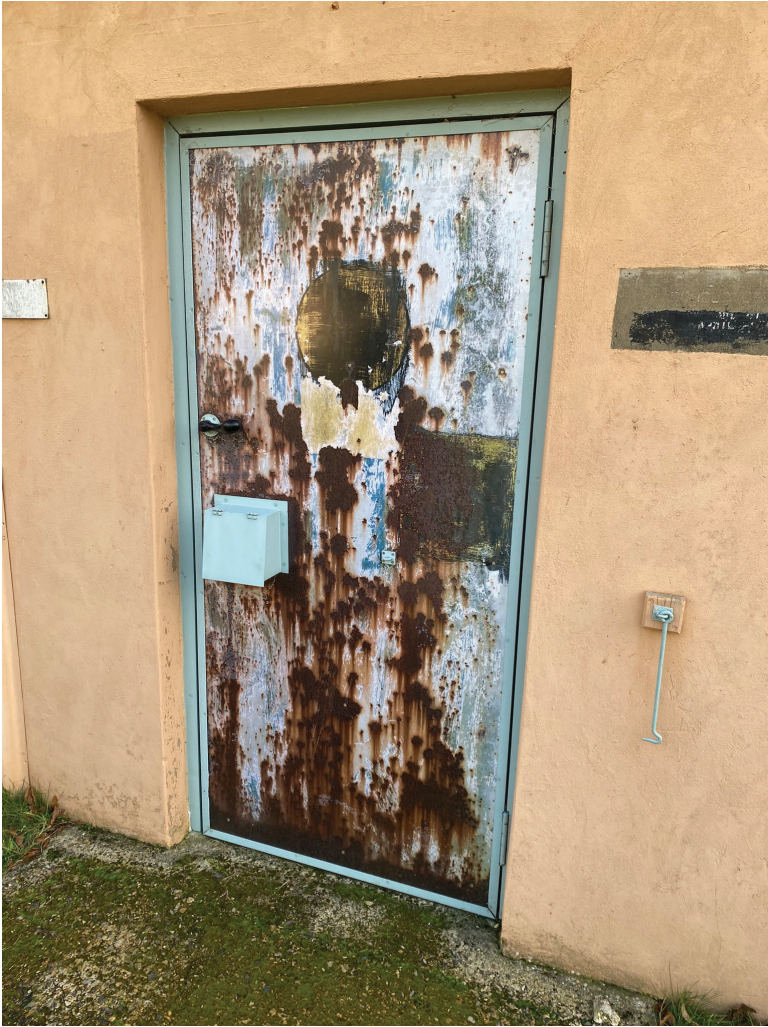
Figure 14.1 Replica vinyl printed door from restoration work at Gorse Industrial Estate (formerly RAF Barnham)
